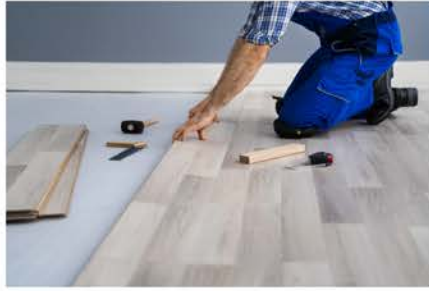
FLOORING INSTALLATION AND REPLACEMENT
