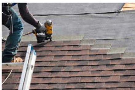
ROOF REPAIR AND REPLACEMENT
