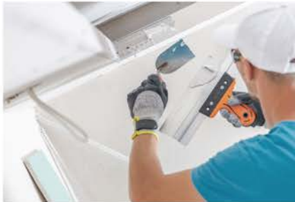
DRYWALL INSTALLATION AND REPAIRS
