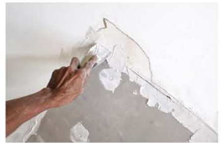
WATER DAMAGE REPAIR
